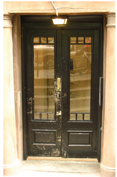
Air leaks. Older doors that have experienced daily use are likely to be worn down and dented, allowing air to leak in and out. Wooden doors like the one showed here are especially susceptible to degradation from moisture, snow and de-icing practices, and daily use; they should be maintained regularly for optimum insulating performance.
