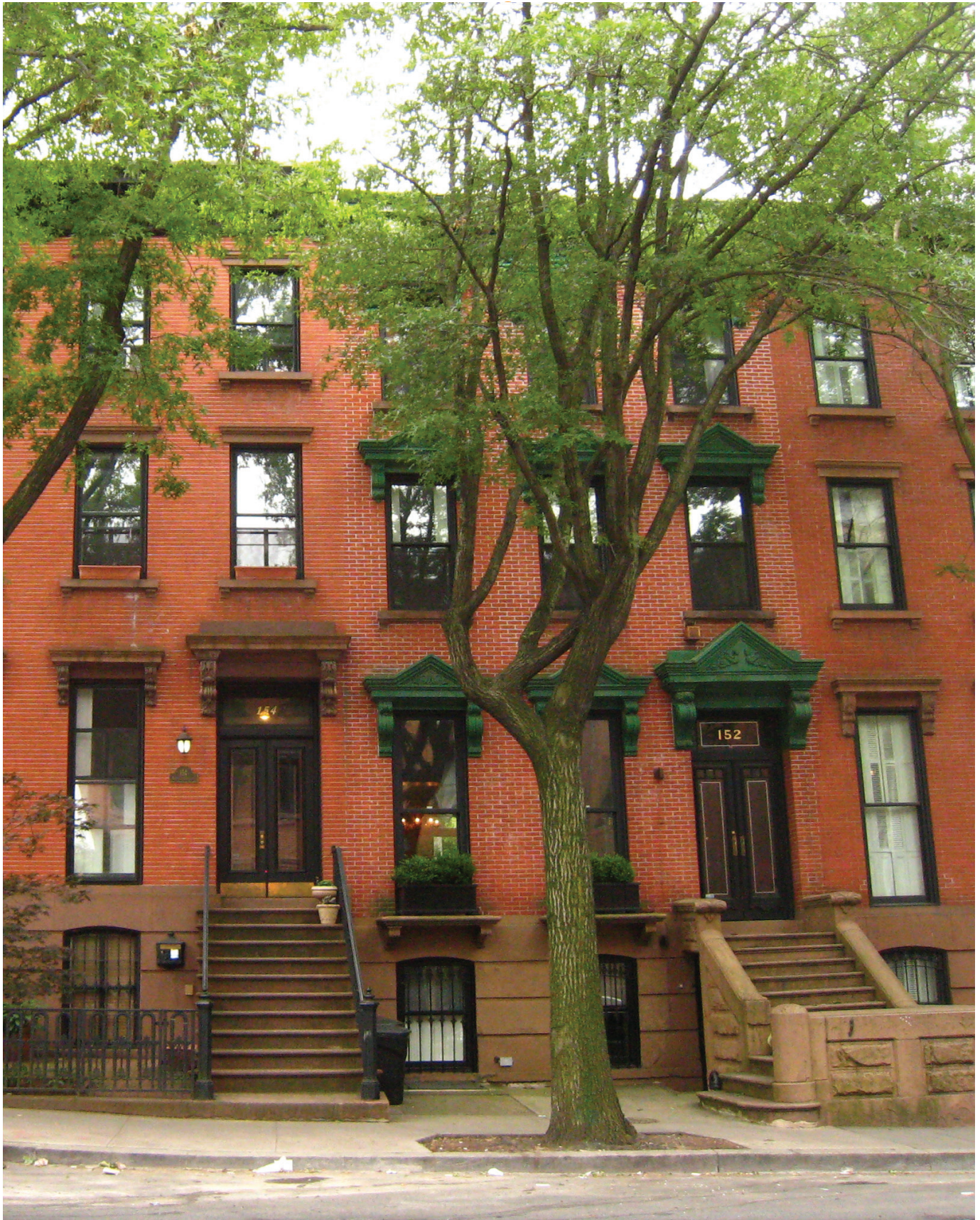
Lafayette Street Rowhouses, Fort Greene Historic District, Brooklyn
