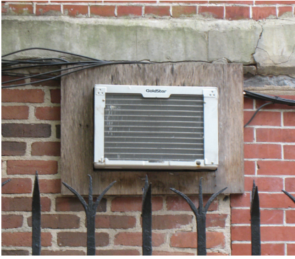
Window AC unit. This poorly installed air conditioner is not properly insulated and will leak air back into the building.
